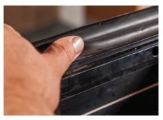
17. To check it is fitted correctly, carefully lift up the edge, checking along the length for bulbous areas that haven't been tucked into the retainer.
