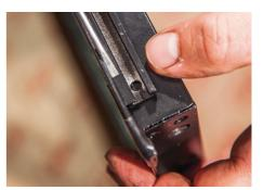
14. On the lower edge, fit the rubber seal retainer with screws or rivets. The deeper return (indicated with screwdriver) should face the outside edge.
