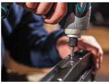
13. Work transfers to the new tailgate. Start by fixing the drain channel to the top. The vertical return should be on the inside edge.
