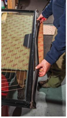
16. To refit the seal, tuck in either end, then the middle. Then, half the distance and tuck that in. Repeat until all is secured.
